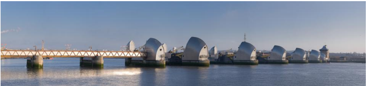
The Thames Barrier from the north bank of the river at Silvertown, in normal (open) operation
