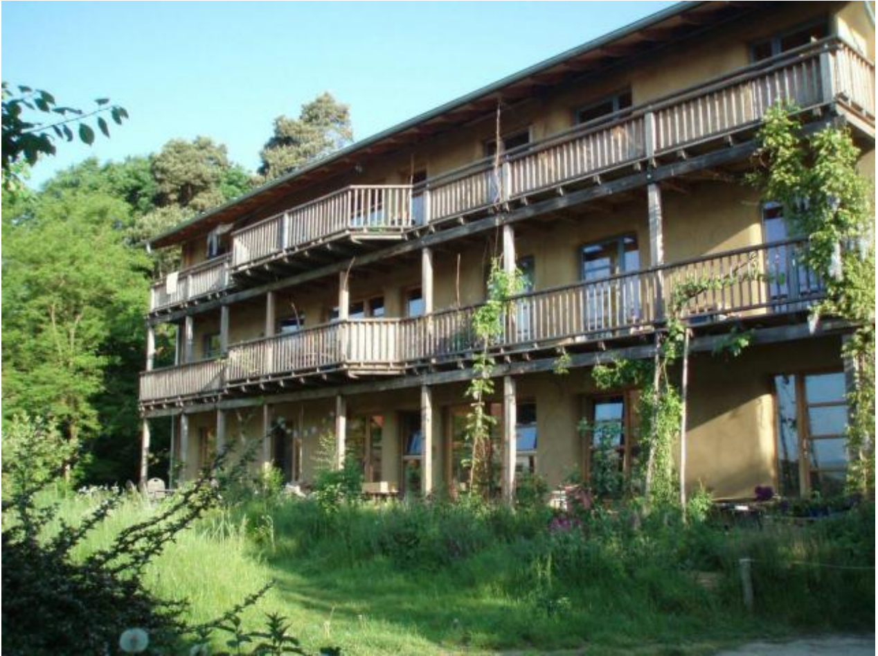
The 'Strohpolis' house in the ecovillage of Sieben Linden - Europe's largest house made out of bales of straw
