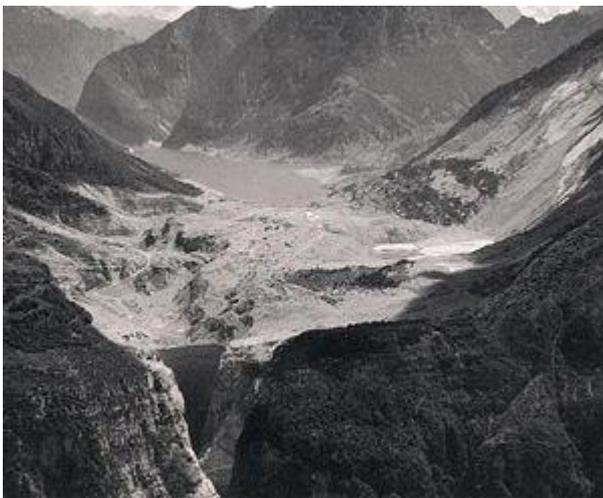
View of the Vajont reservoir after the landslide (1963).
