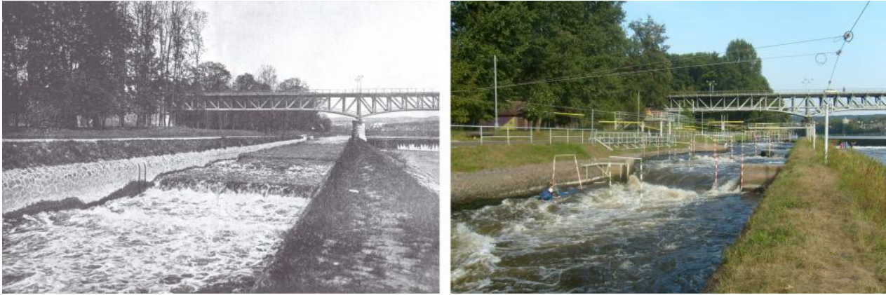
Comparison of the raft sluice in Raudnitz 1912 (left photo) and the situation in 2009 (right photo)
