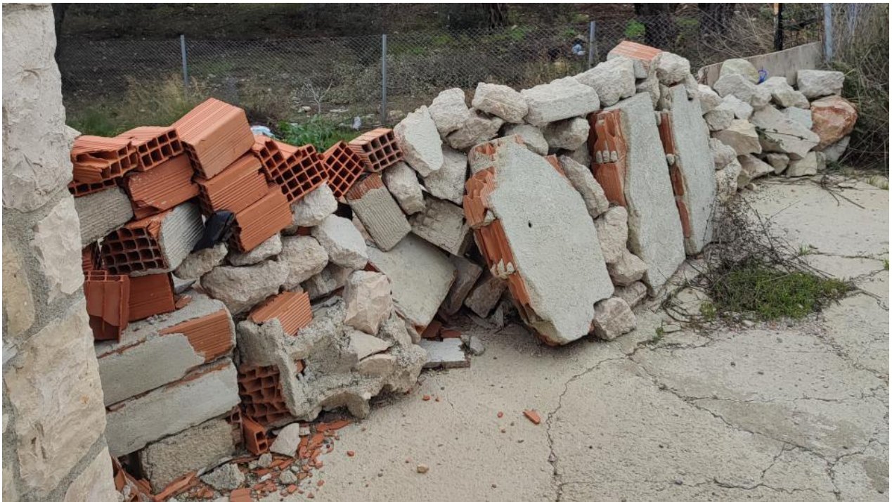
Makeshift wall to keep the boars out of a small artichoke field in İncik village.
