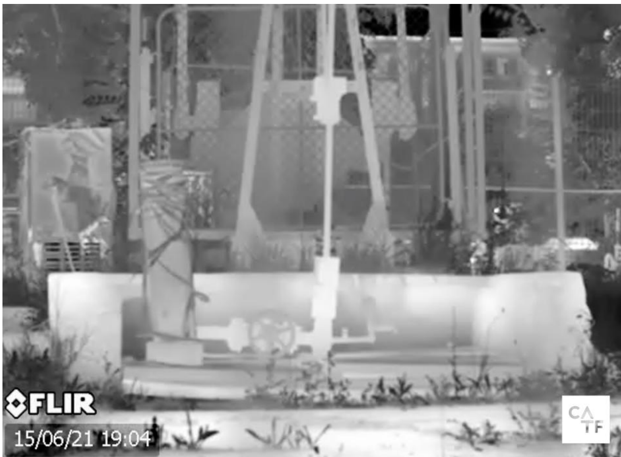
Infrared picture of leaking methane well in Câmpina, Prahova County, Romania.
