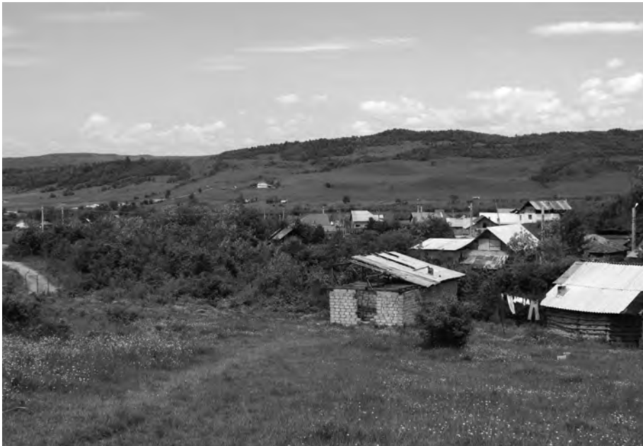
Figure 2: Construction of houses in Drago- miresti.
