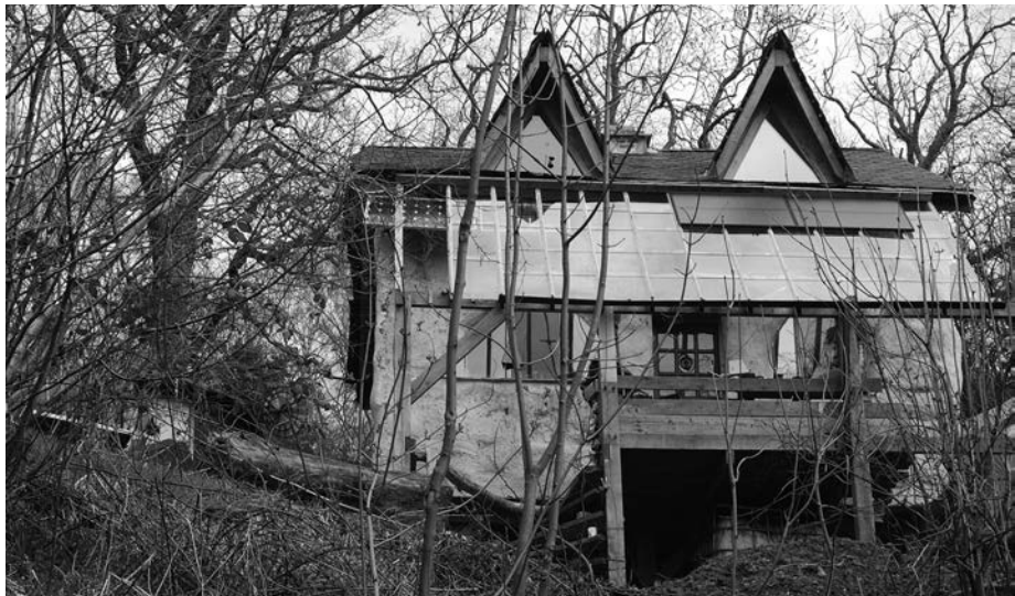
Figure 1: An eco-house in Green Hills, Scotland
