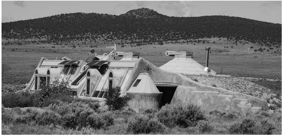
Figure 4: Earthship in the Greater World Earthship Community, Taos, New Mexico, USA.
