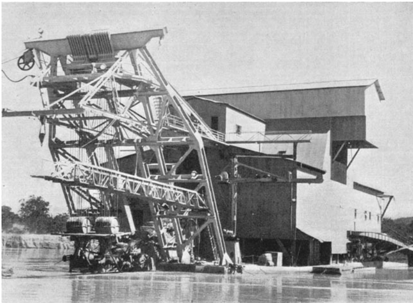
FIGURE 2. 'No. 2 Dredge', Tableland Tin Dredging N.L., 1946. (Source: Queensland Government Mining Journal (47, 21 October 1946): 298.)
