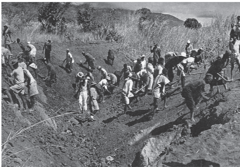
Figure 10.2. Peasants filling in one of the eroded gullies at Domasi in the early 1950s
