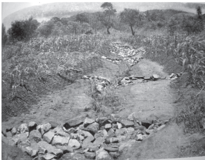
Figure 5.4. Controlling gully erosion with stone check dams, 1953
