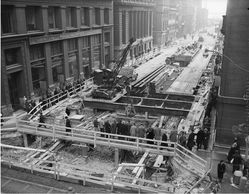
FIGURE 6.1. Cut-and-cover subway construction along Yonge Street, c. 1949. Courtesy of City of Toronto Archives.
