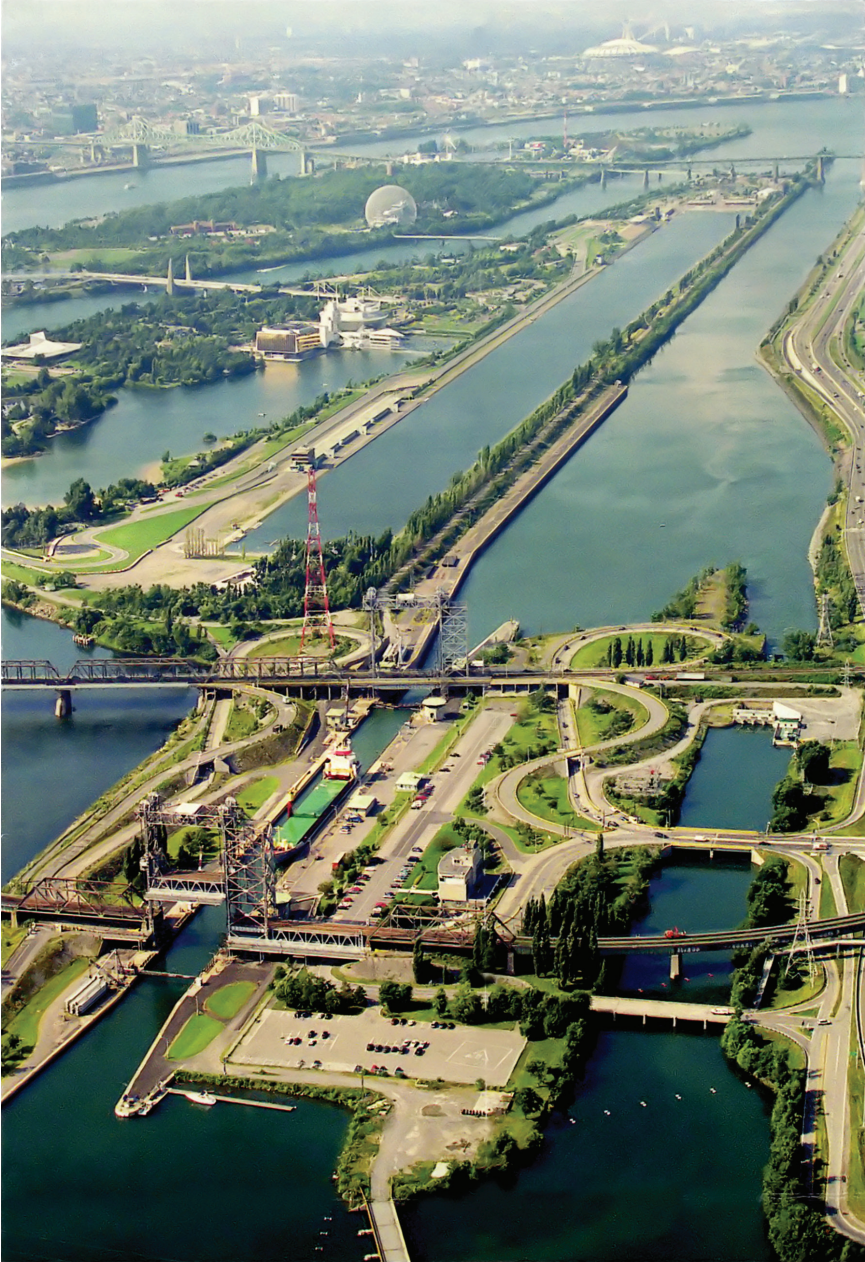
FIGURE 5.6. St. Lawrence Seaway at Montreal. Courtesy of Library and Archives Canada.
