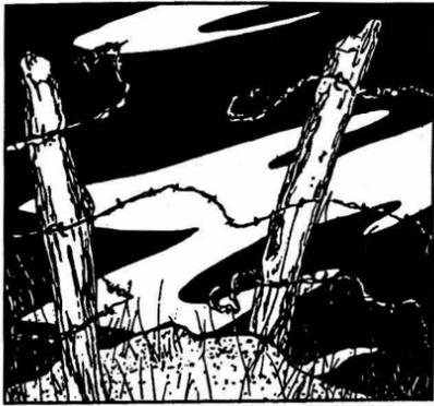
Field fencing topped by two strands of barbed wire is the most diabolical. The strands are often close together and hanging slack—a recipe for disaster. I loosen both strands and tie them to the field fencing, leaving no gaps.
