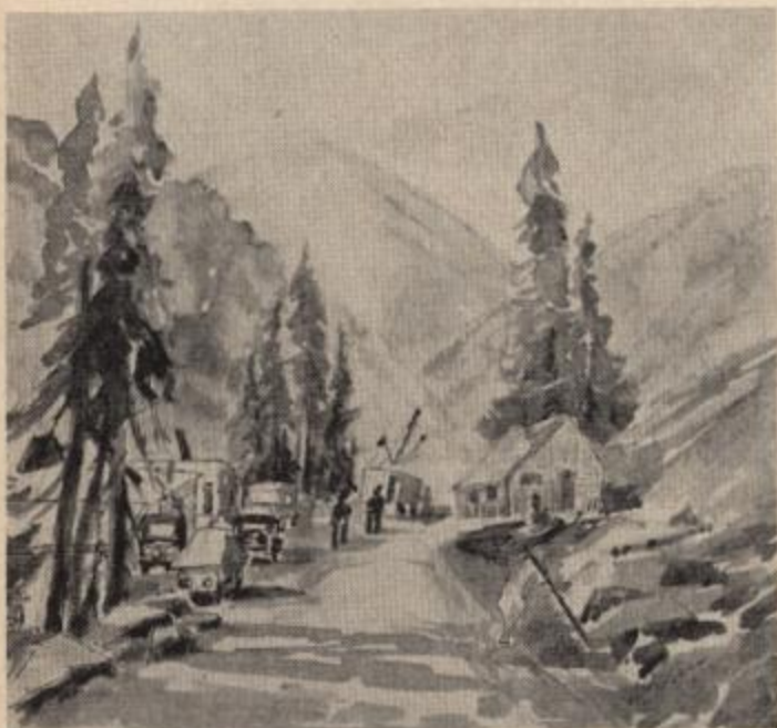
Road Construction Camp
