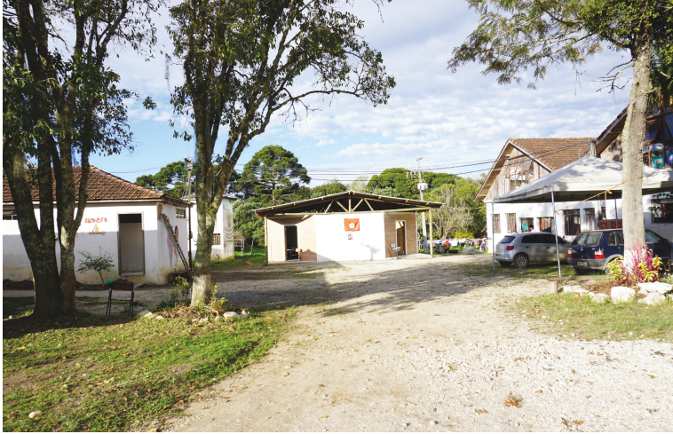
Figure 16: View of ERS's main buildings. Left: dormitories and bathrooms; center: lecture hall; right: offices and dining hall
