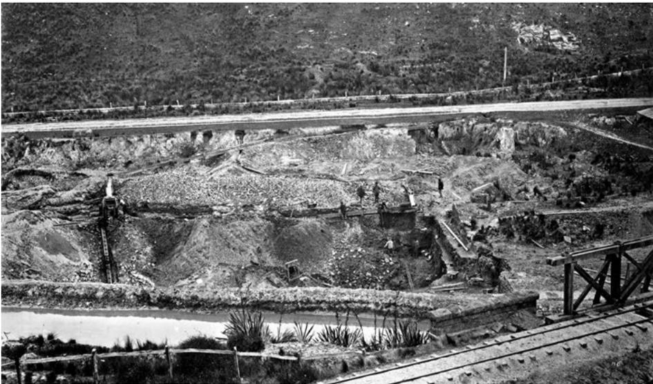
Photo 1: A very rare photograph showing Cantonese miners utilising a Chinese Pump. This is on the far left, in the centre of the image and is being driven by a small waterwheel.
