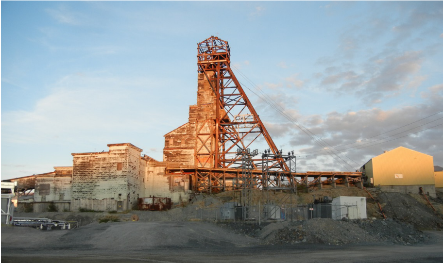
Figure 2: Giant Mine Shaft no. 2 headframe partially deconstructed, July 2012. The mine site is currently undergoing extensive subsurface and surface remediation. Photo by Kevin O'Reilly.
