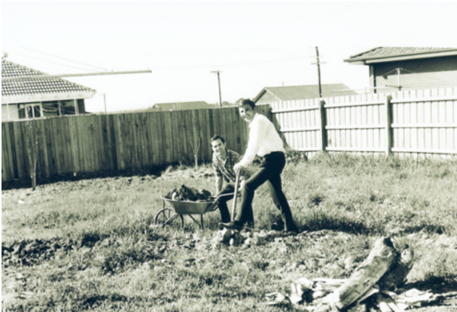
The author's father, Steve Zelko (left), and his friend and fellow Yugoslav refugee, Karol Grah, begin digging the foundations for a new suburban house (courtesy of the author).
