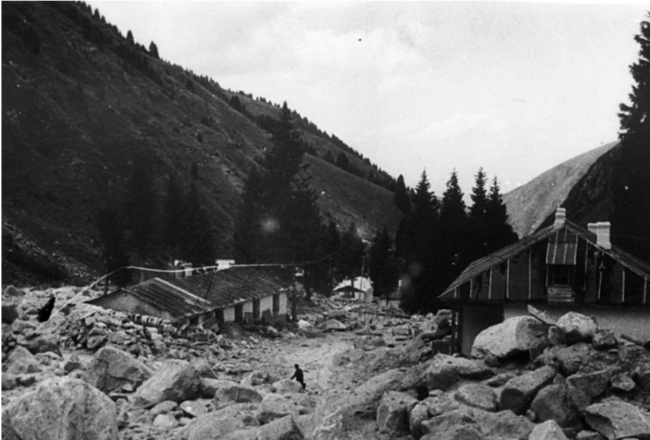
Houses covered with rocks after a mudflow in Malaia-Almatinka Valley, Kazakhstan, 1956 (Source: Central State Archive, the Republic of Kazakhstan, 2-46946).
