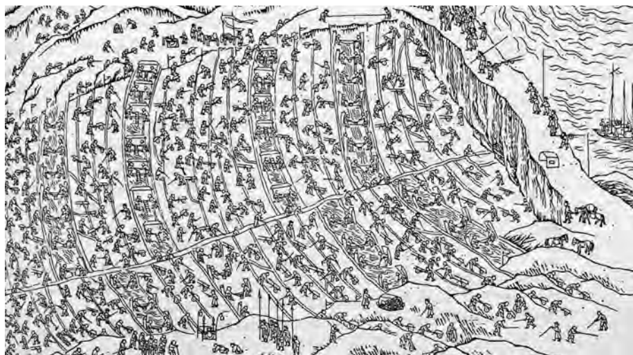
Figure 9: Drawing (1833-42 AD) by hydraulic engineer Lin- Chhing, showing the organization of labor during the cutting of a canal (Needham, Science and Civilization in China, vol. 4, part III, 262)
