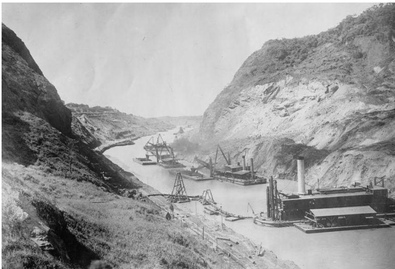
Photo of the dredges removing material from the Cucaracha slide in the Culebra Cut, ca. 1913.
